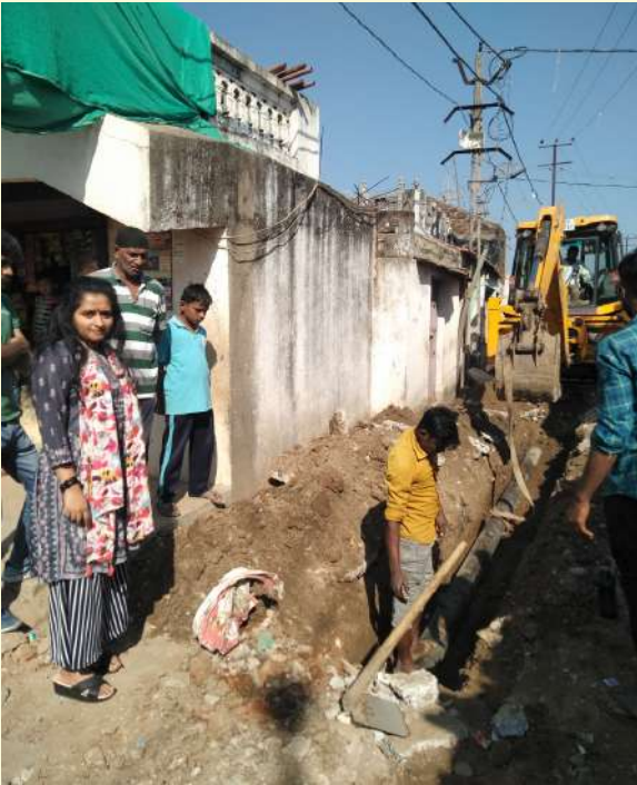
Intern doing inspection at Construction site, Vadodara, Gujarat
