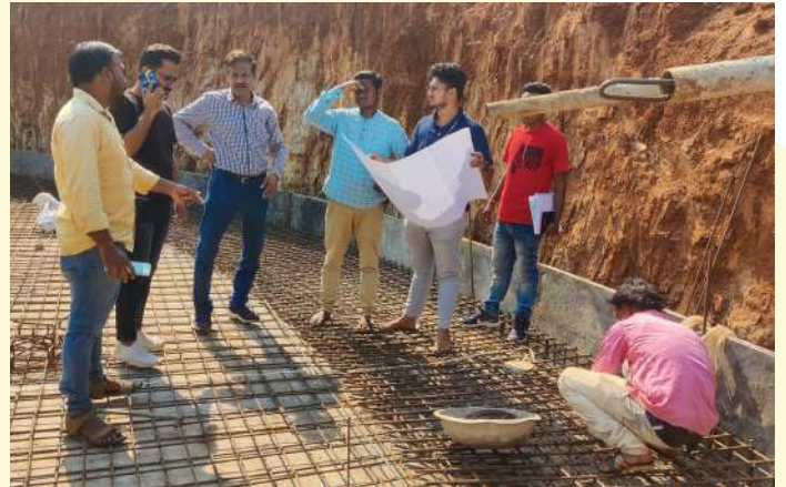
Interns working at site Rayagada, Odisha
