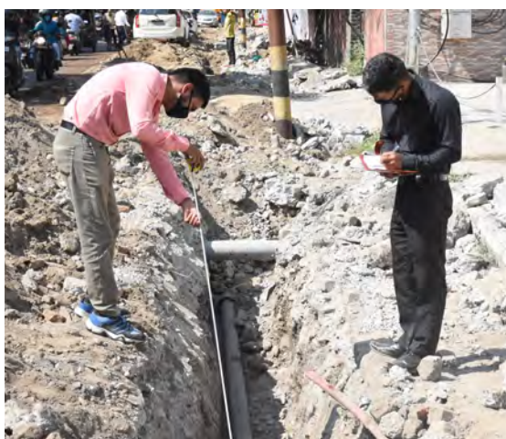
Dehradun Smart City intern measuring the excavation depth of the distribution of the main pipeline under the Smart Road Project.
